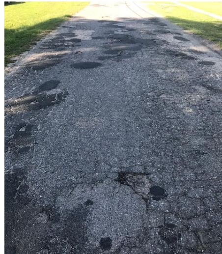
East St.- Cracked road and potholes.
