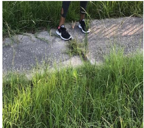
Cannon St. - Near 2 yellow houses with black fence. Raised/uneven and crack sidewalks (other view).
