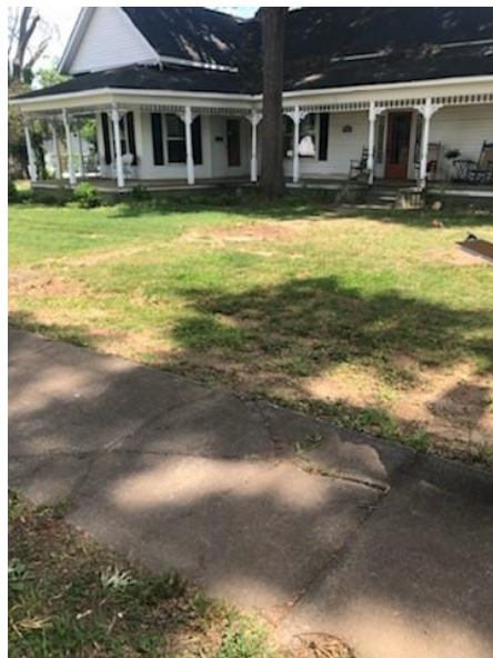
In front of Rowell House: Cracks in sidewalks/Dip in sidewalk and incline
